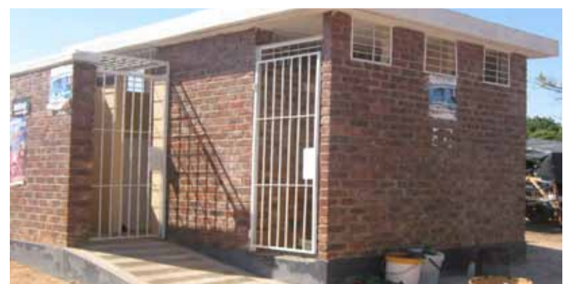
A harvest by Budiriro 1 Primary shows how they are making use of the borehole constructed under the CDF. Middle: The footbridge that links Budiriro 2 and 4. Below: The toilets at Budiriro 4 Shopping Centre
