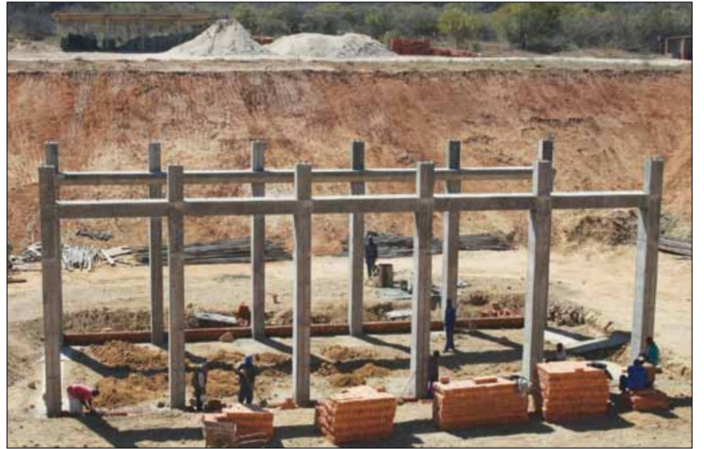
Mtshabezi main pump house under construction
